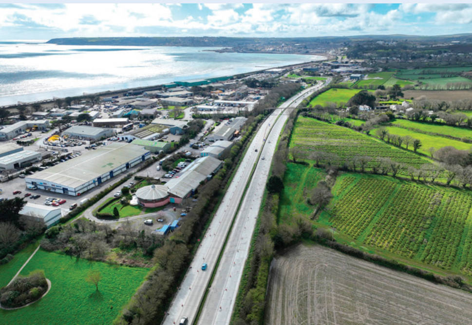
Next Generation Concrete Surface was trialled on the A30
