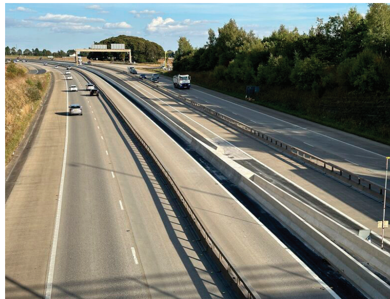
Rigid concrete barriers are robust enough to contain heavy electric vehicles
